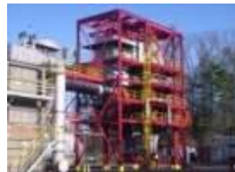
Alstom BSF Windsor US - 15 MWth Oxy - Coals
