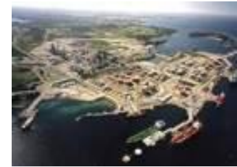
Statoil Mongstad Norway - 40 MWth Chilled Ammonia - Gas
