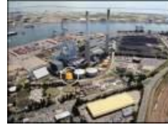
EDF - Le Havre France - 5 MWth Adv. Amines - Coal
